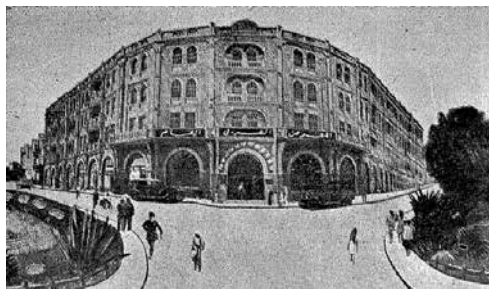
Figure 4. "The view of the Awqaf Hotel, the building where the exhibition is taking place, built according to the glamorous Arab style. It is four stories high and cost no less than ninety thousand Palestinian Pounds and used to be leased for eight thousand pounds annually." Source: al-'Arab , 15 July 1933, 22.
