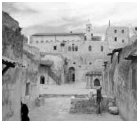
Figure 2. Ethiopian monks' rooms on the roof of the Holy Sepulcher.
