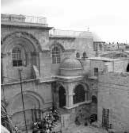
Figure 3. Stairs from roof to portico.
