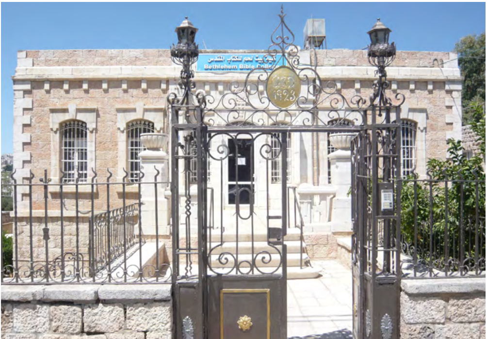
Figures 10 and 11. The houses built by Mikhail Dabdoub and Jubrail Dabdoub on Hebron Road, Bethlehem, in 1922 and 1923.
