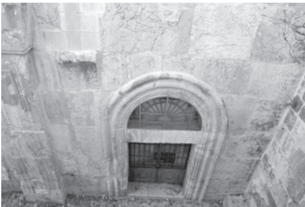
Figure 15: South entrance of the Golden Gate from the south. Detail shows the springing of an arch to the upper left of the entrance. Source: St. Laurent, 1993.
