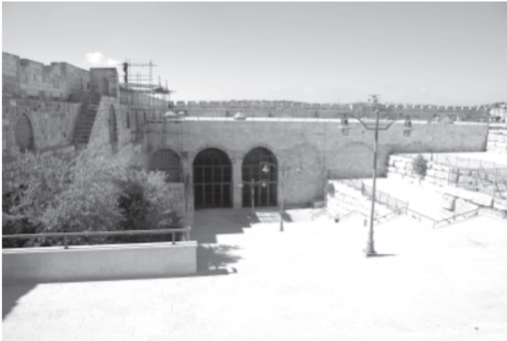
Figure 13: North portal façade from the north. Source: St. Laurent, 2012.
