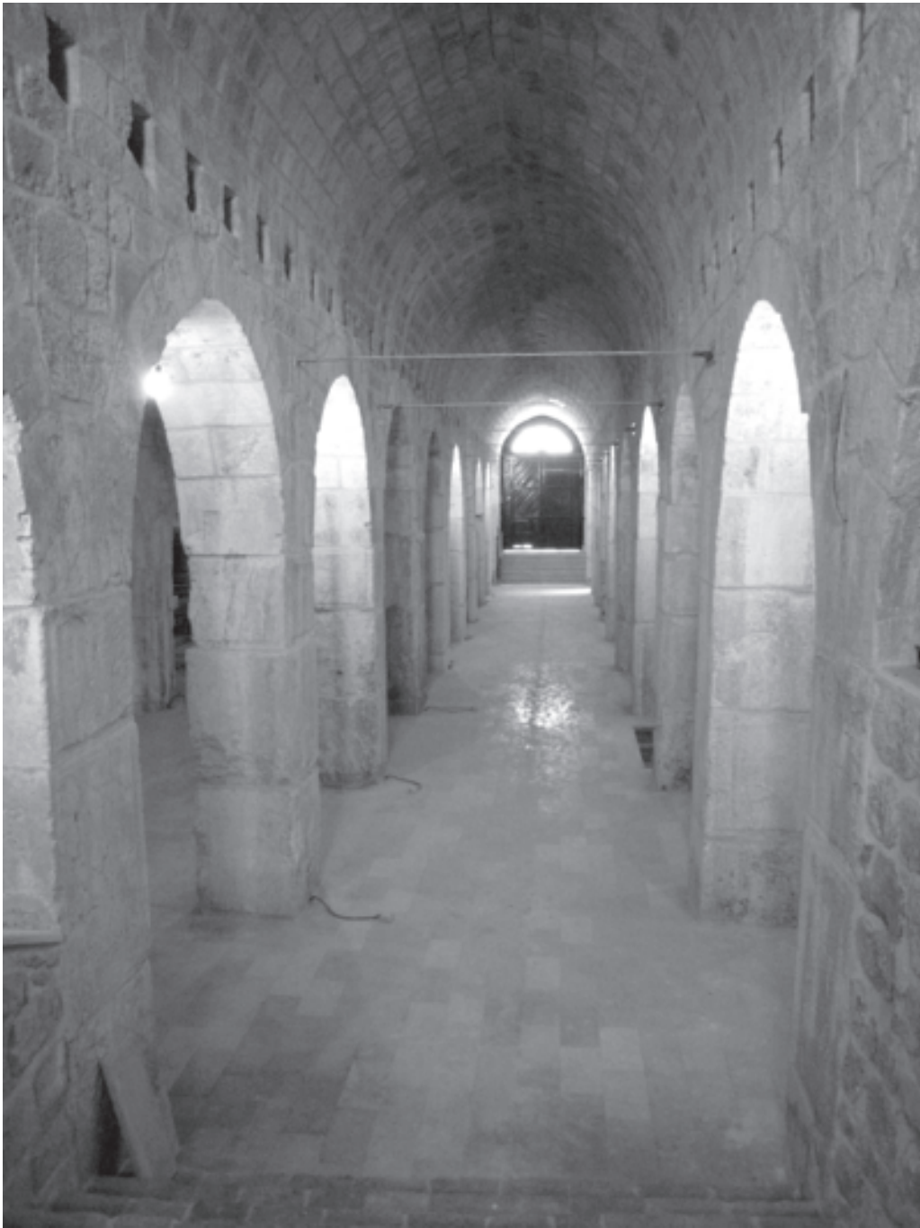
Figure 3: Interior of the Mosque of Mu'awiya showing aisle 4 and the piers of re-used Herodian stones. Source: St. Laurent, 2007.
