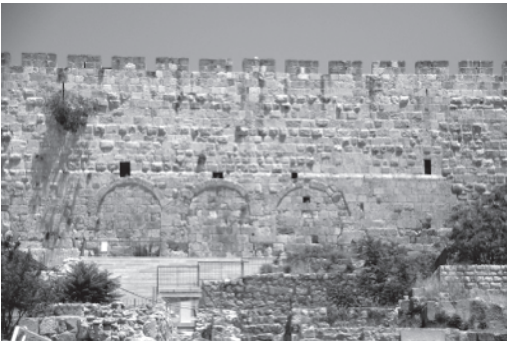
Figure 7: Triple Gate showing arch construction. Source: St. Laurent, 2012.
