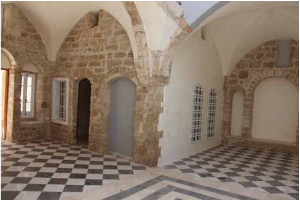
Figure 3. The central hall of Dar al-Ghusayn after restoration, Gaza City, 2020. RIWAQ photo archives.
