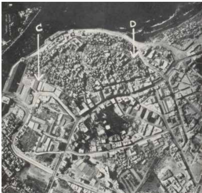
Figure 5. Two aerial photographs of Jaffa that appear in a 1938 British report, captioned “Demolitions completed on 18 June between points A and B,” and “The second stage of Demolitions – The circular road C-D completed on the 20/30. June” in “Military Lessons of the Arab Rebellion in Palestine 1936,” (1938) IOR/L/MIL/17/16/16, British Library, India Office Records and Private Papers.
