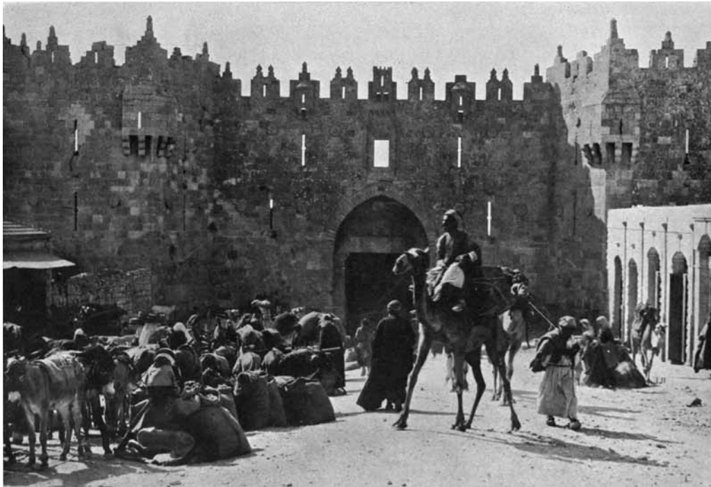
Fig. 4: Commerce at Damascus Gate, 1918-1920. A photograph selected by Ashbee of a view of Damascus Gate from outside the Old City at some time between 1918-1920. The image shows commercial buildings were constructed right up to the Old City walls either side of the gate; A busy commercial scene including Bedouins is shown in the foreground. Source: Illustration 7 from Jerusalem, 1918-1920. London, J. Murray.
