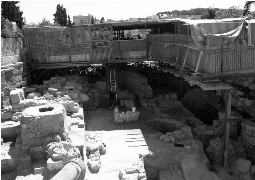
Fig. 3: Area slated for development above excavations area by visitors' centre. Source: Conflict in Cities.
