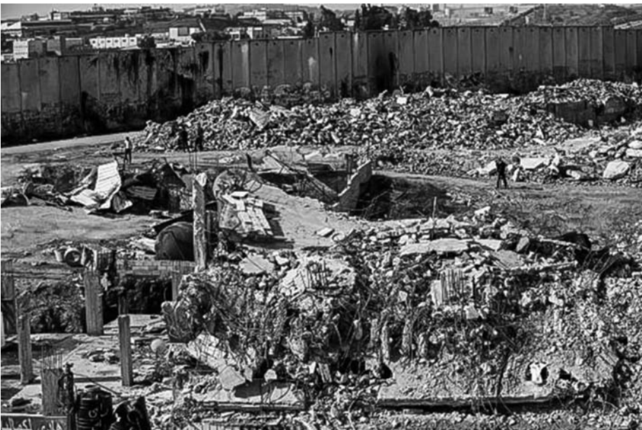
The demolished remains of the three-story home belonging to the family of Ali Khalifa, who was killed by Israeli forces in 2011. The Qalandia residence, which continued to house Khalifa's family, was evacuated before being demolished by the Israeli army. (23 October, Ahmad Gharabli/AFP via Getty Images)
